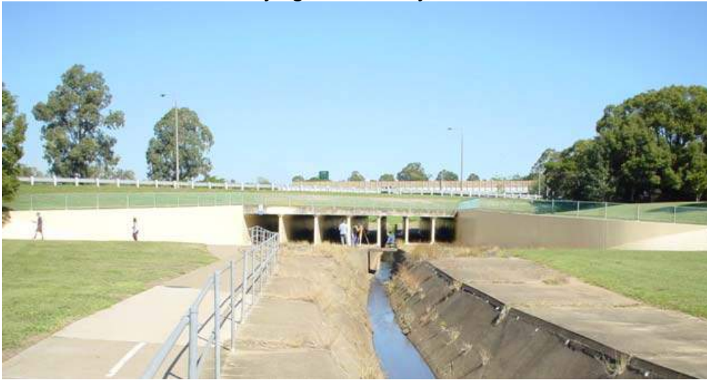
Fig. 2 - Photographs of a Minimum Energy Loss culvert in Brisbane ( Q_{des} = 220 \text{ m}^3/\text{s} , B_{max} = 42 \text{ m} , B_{min} = 21.3 \text{ m} , D = 3.0 \text{ m} )
