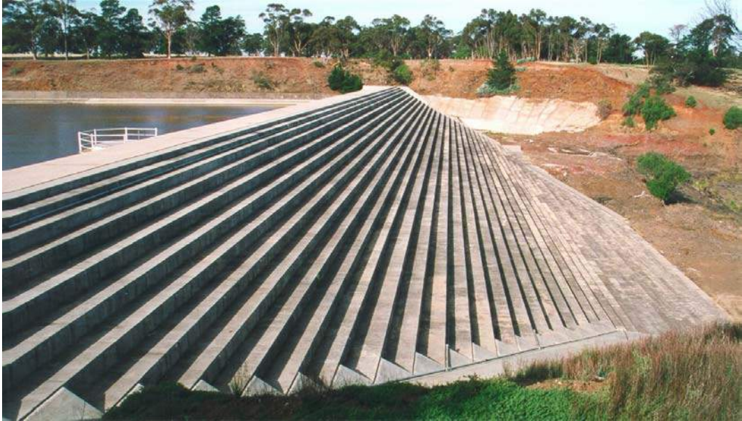
Fig. 3 - Melton dam stepped spillway on 30 January 2000 - Completed in 1916, the Melton dam was equipped in 1994 with a secondary stepped spillway ( Q_{des} = 2,800 \text{ m}^3/\text{s} , h = 0.6 \text{ m} )
